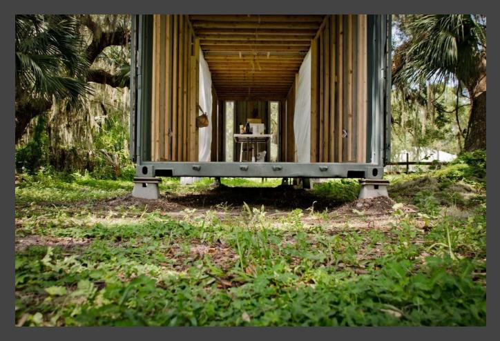
I regularly monitor the leveling of the container and often inspect the bottom of the structure for deterioration. After one year, it still looks great. I also think the spray foam insulation on the bottom helps to preserve the structure (against humidity and rust). So far, no exotic critters have established their home under there.
