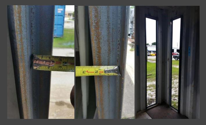
The same system was used for the two large sliding doors on each side of the container. Each of those sliding doors is 10 feet wide by 8 feet high and are enclosed in an aluminum frame. The large sliding doors are made of double pane tempered glass, without Low-E treatment (Low-E can form streaks after a few years: bad!). The sliding doors are also installed from the inside and their aluminum frame is pushed and glued with silicone against the steel frame.
