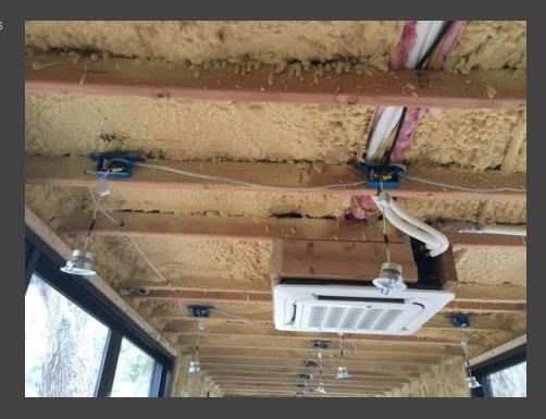
day, the cooling unit works constantly. I do not recommend a smaller unit, a couple more thousand BTU would be better. The indoor unit connects to the outdoor unit via a conduit running along the ceiling which exists through the back wall of the container. I was told to never drill a hole in the roof of a shipping container, and I am glad I followed this advice.
